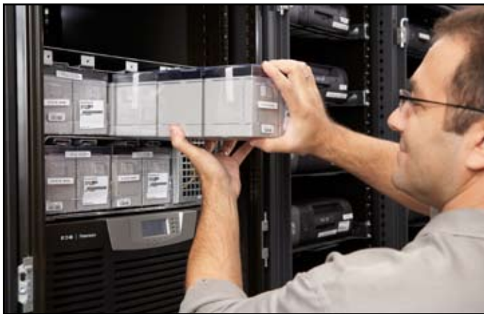
IT staff can easily replace battery modules.
